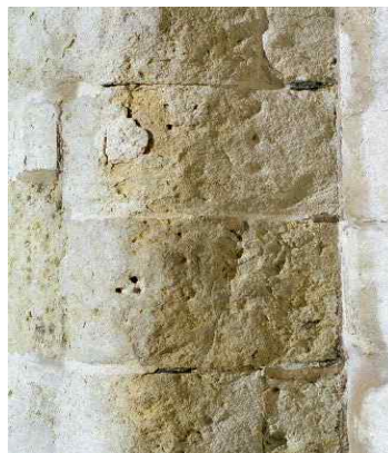
Fig. 4.6 – Stone masonry damaged by freezing
