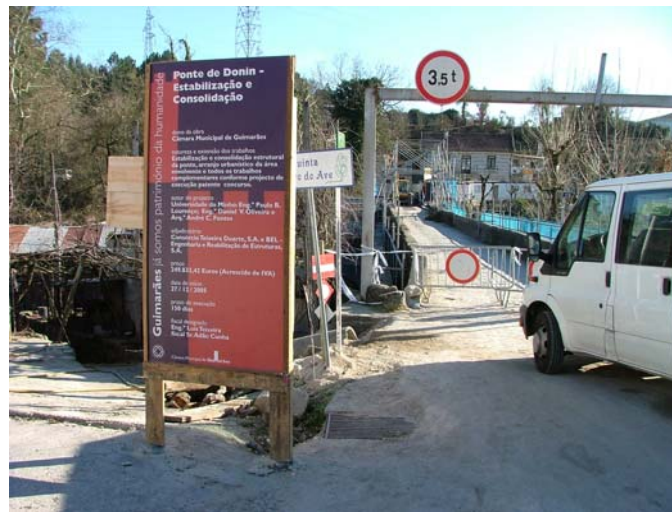
Fig. 6.6 – Blocked access on the bridge
