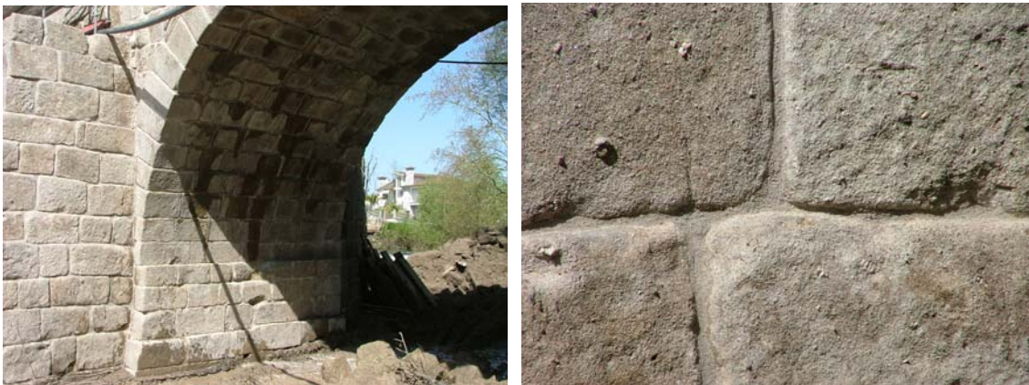
Fig. 6.26 – Joints repointed with sand-lime mortar matching the colour of the stones
