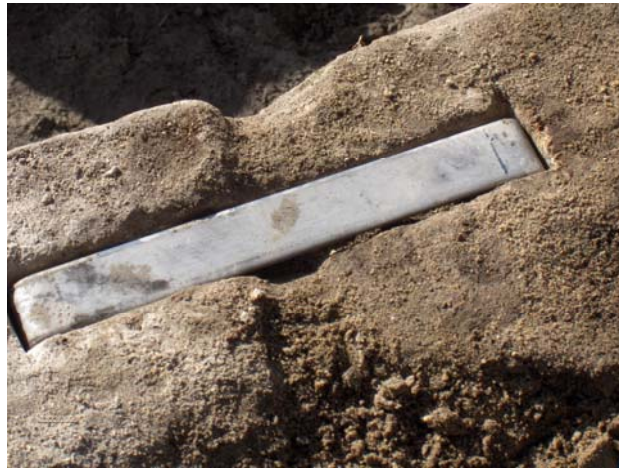
Fig. 6.23 – Stainless steel cramps
