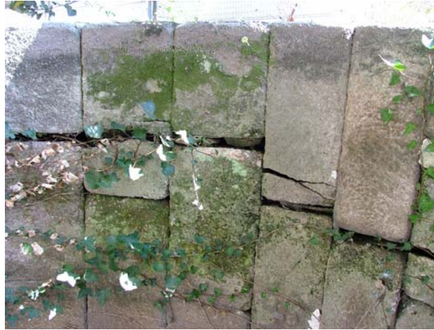
Fig. 4.4 – Splitting beneath the spandrel walls
