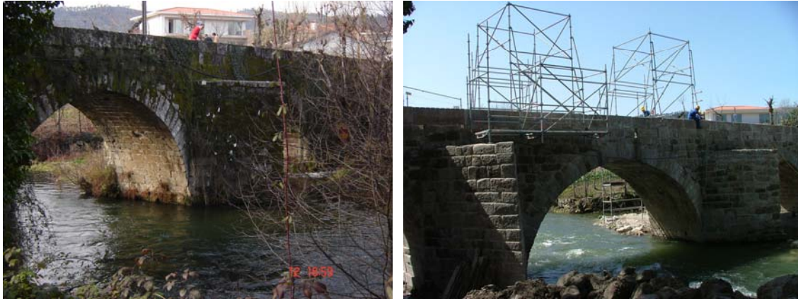
Fig. 6.25 – Donim Bridge before and after the removal of vegetation
