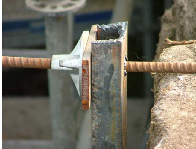
Fig. 6.14 – Tie bars – Restrain mechanism
