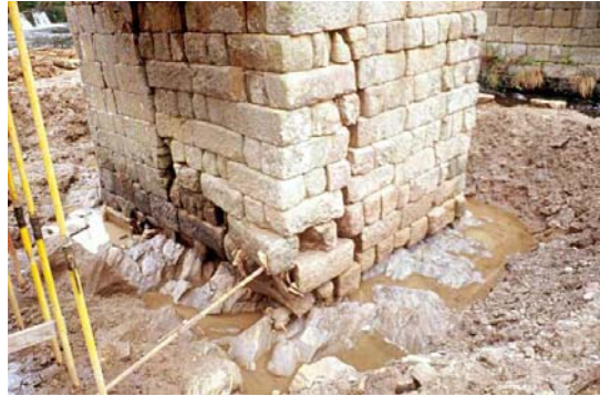
Fig. 4.3 – Damaged foundation
