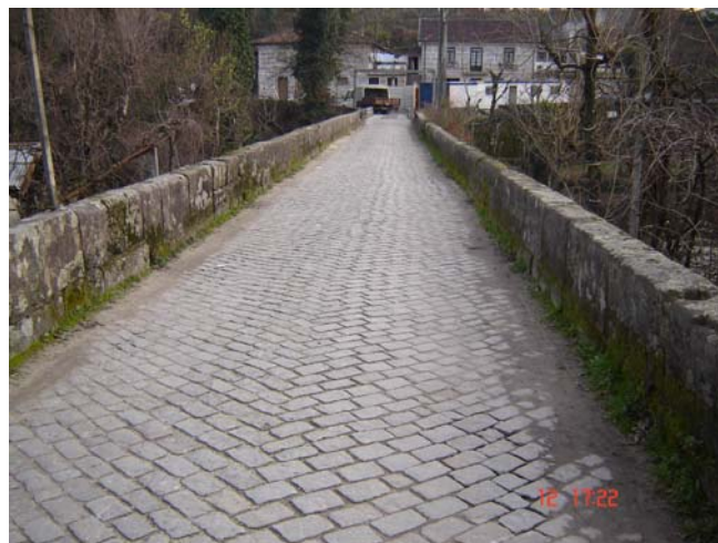
Fig. 6.1 – Donim Bridge – Road way
