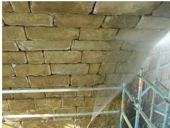
Fig. 6.24 – Spraying biocide
