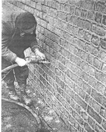
Fig. 5.1 – Repointing of the joints
