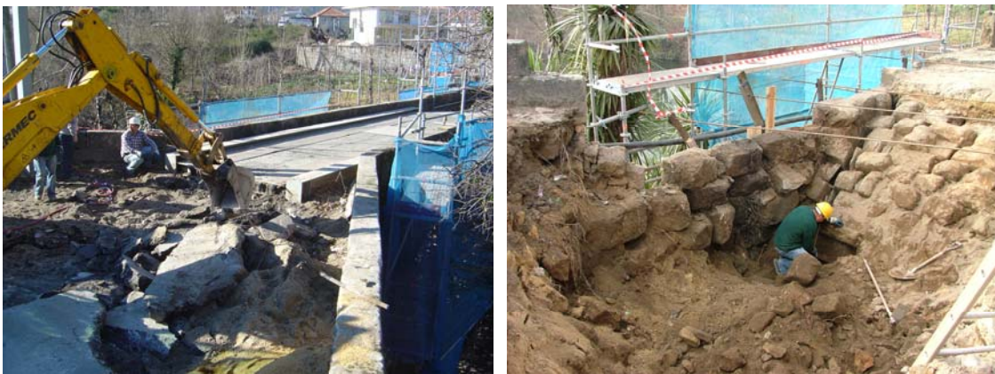
Fig. 6.15 – Excavation of the fill material:
