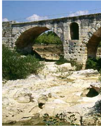
Fig. 1.5 – Flood opening in pier
