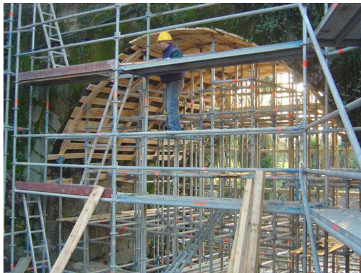
Fig. 6.11 – Propping the arch A1
