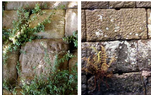
Fig. 4.7 – Stone masonry affected by plant growth
