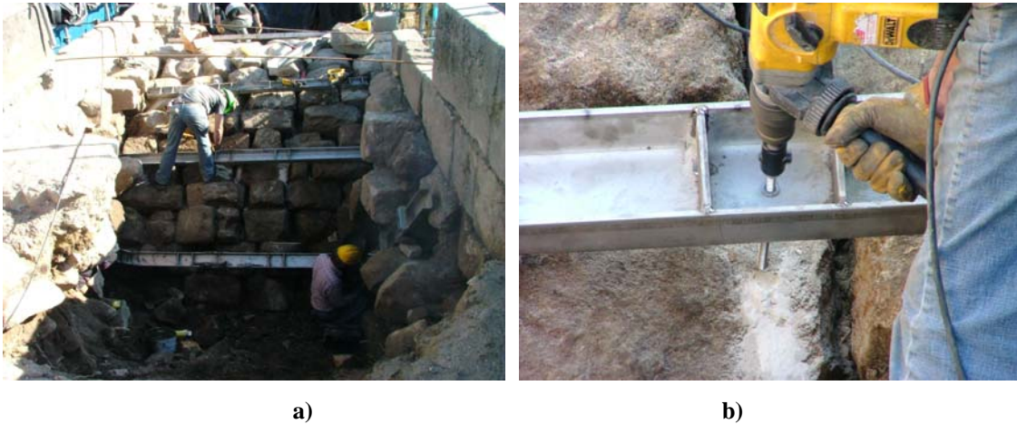
Fig. 6.18 – Repairs on arch A1 a) Metallic profiles; b) Drill for the stitching anchor rods
